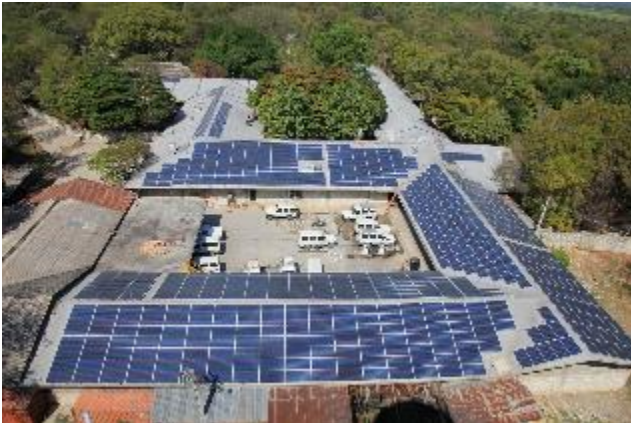
Figure 7: The installed PV plant on the roof of the clinic.
