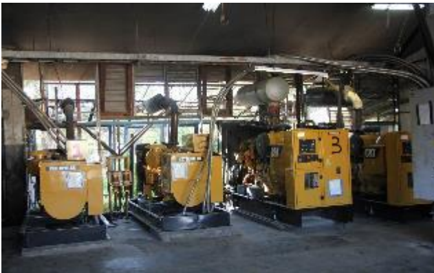
Figure 8: The four diesel genset of the off-grid system.
