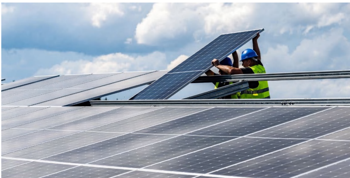
Figure 48: Solar installers at work in Langenenslingen-Wilfingen in 2024 © EnBW Uli Deck
