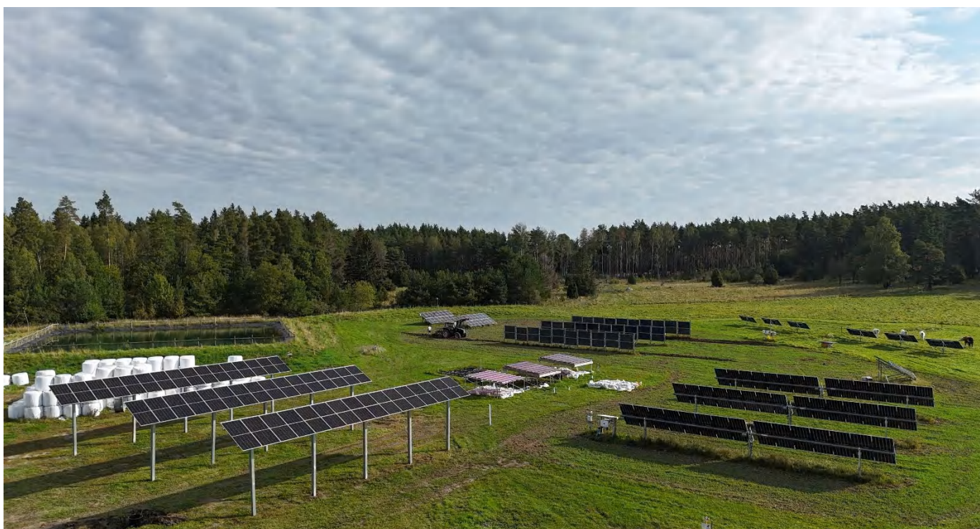
Figure 54: Agrivoltaic system with bifacial photovoltaic modules installed at Kärbo Prästgård, Västerås, Sweden (Source: SOLVE).
