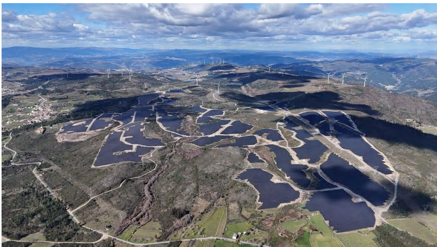
Figure 42: Solar PV power plant “Douro”, in Vila Chã da Beira, Portugal, owned by Sonnedix, has a capacity of 150 MW and started operation in 2025.
