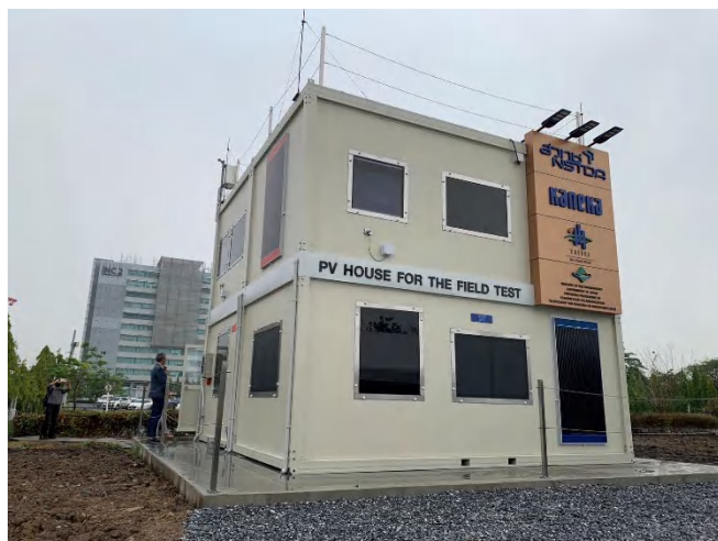
Figure 61: BIPV Demonstration at NSTDA.
