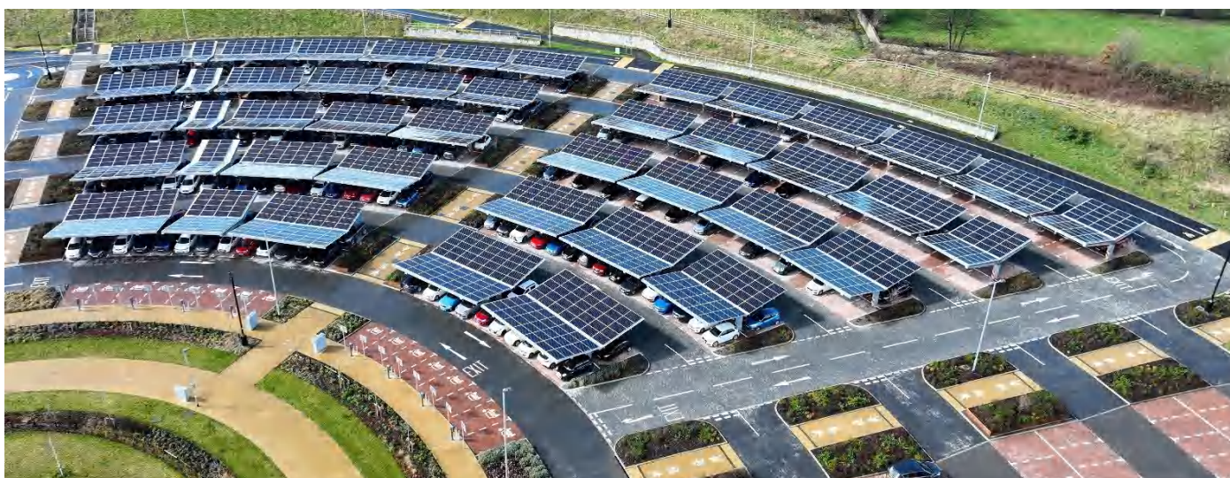
Figure 63: The Stourton Park & Ride, which opened in 2021, is the first solar carpark in the UK, with 1.2MW solar, 500kW/950kWh battery system and 26 EV charging units.
