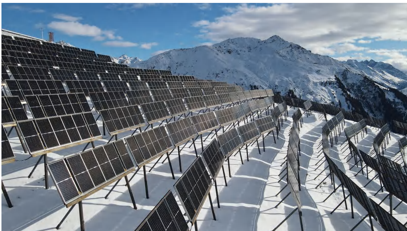
Figure 56: «Madrisa Solar», Switzerland's first alpine large-scale photovoltaic plant located at around 2 000 m above Klosters, began feeding electricity into the grid in 2025 as part of the national «Solarexpress» (EKZ / Repower, 2025). Currently, about 15% of the installation is connected. Once fully built, the project will comprise approximately 20 000 bifacial modules of 580 Wp each, corresponding to an installed DC capacity of around 11 MWp. By 2027, the plant is expected to produce around 17 GWh annually, over 40% of it in winter, thus contributing to Swiss winter electricity supply. The total investment amounts to approximately 70 million Swiss francs (Photo: Madrisa Solar AG).
