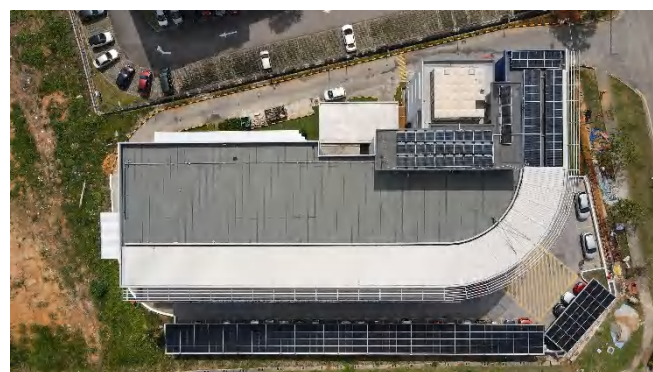
Figure 33: Aerial view of SEDA Malaysia building with rooftop and car park solar PV installations.
