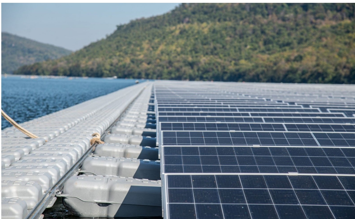
Figure 60: 24 MW EGAT's Hydro-Floating Solar Hybrid located in Khon Kaen province, Thailand.
