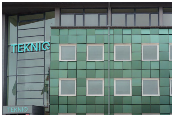
Figure 11: SolarLab 98.9 kWp BIPV plant at TEKNIQ Headquarters in Glostrup showcases a full-façade upgrade that combines refined architectural expression with high-performing, integrated photovoltaics.
