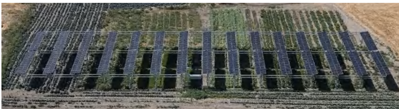
Figure 62: Ayaş AgriPV Facility, Ankara: An exemplary application achieving dual land-use productivity through the integrated use of solar panels and agricultural areas.
