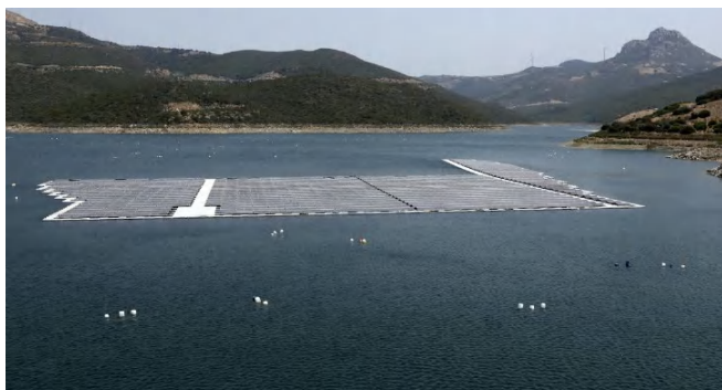
Figure 35: Floating park 13 MW in Oued Rmel, Tangier (Ref: h24)
