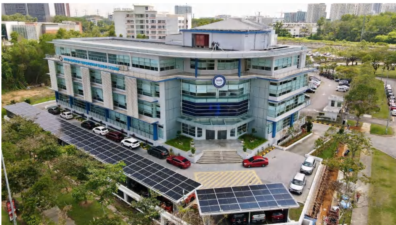
Figure 32: SEDA Malaysia new office building featuring rooftop and parking canopy solar PV installations to support on-site renewable energy generation.
