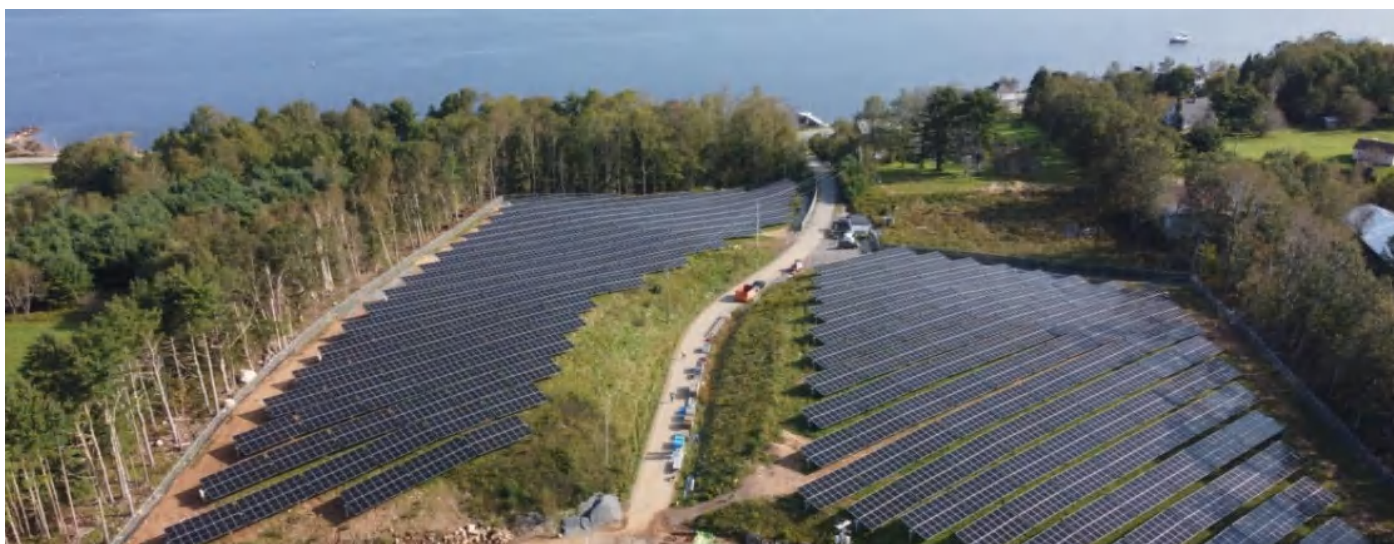
Figure 8: Inaugurated in January 2024, the 4.8 MW community-owned PV array in Mahone Bay, Nova Scotia, is part of the province's Community Solar Program which facilitates shared ownership of PV projects. The array was partly funded by the Government of Canada and the project was developed by AREA, a 100% municipally owned company formed in 2014 (photo credit: Goldbeck Solar).
