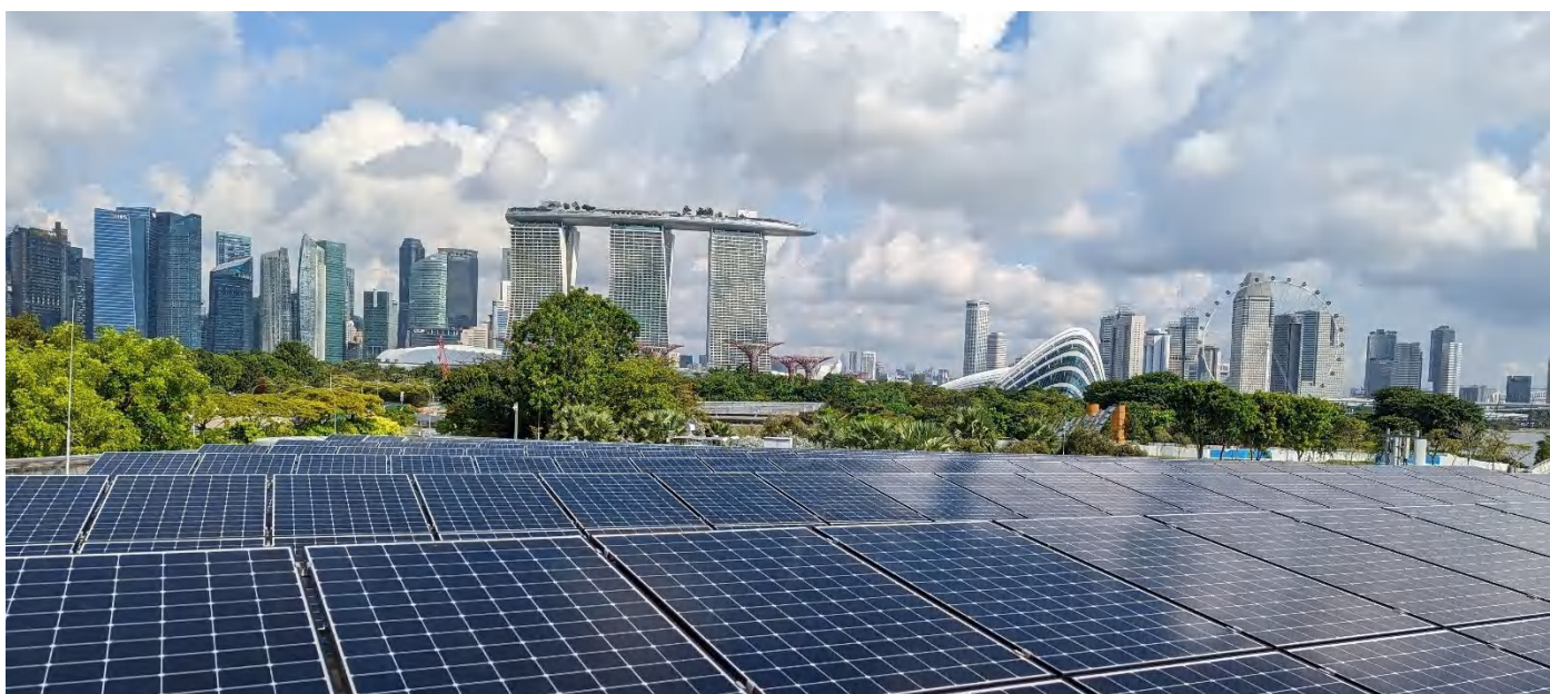
Figure 45: Singapore strives to strike a balance between green and solar: this site is a test system from SERIS exploring impact of climate on energy yield.
