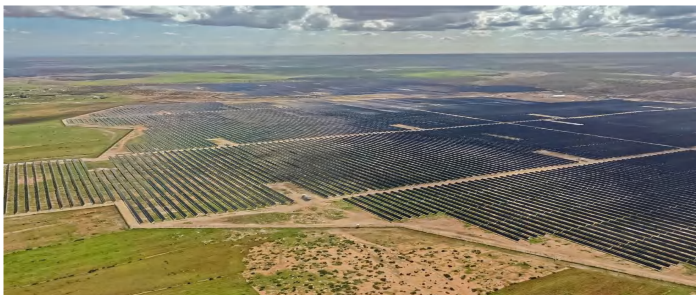
Figure 34: Largest PV plant in Morocco, Khouribga. Ref : https://www.infomediaire.net/ocp-green-energy-premiere-phase-programme-solaire-202-mwc/ .
