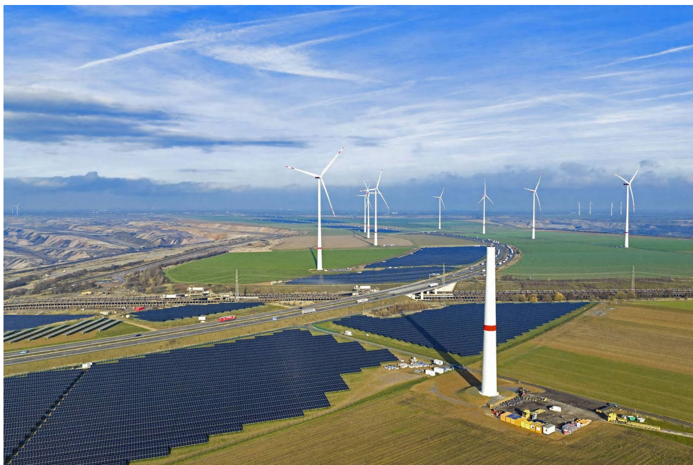
Figure 17: Photovoltaic system at open-cast mine in North Rhine-Westphalia (© RWE).
